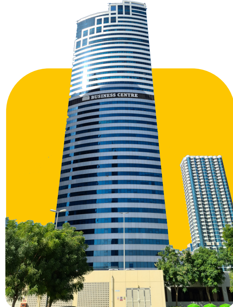
HDS BUSINESS CENTRE JUMEIRAH LAKES TOWER
