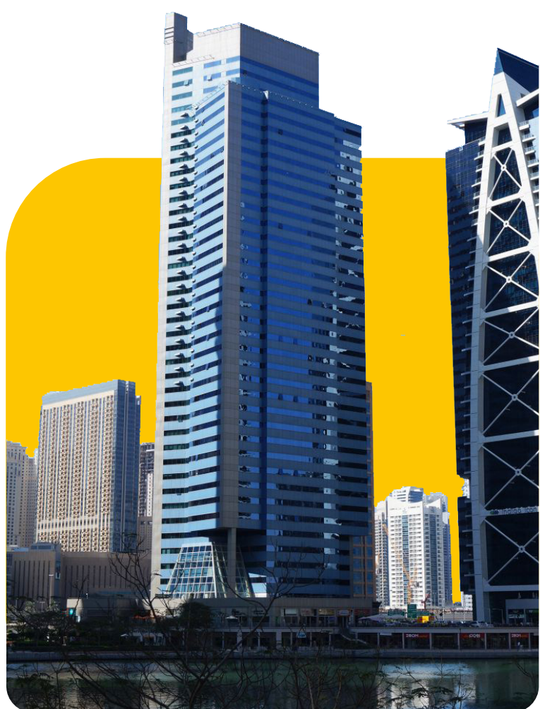
HDS TOWER JUMEIRAH LAKES TOWER
